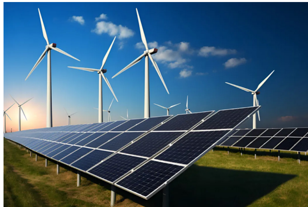
风力发电与光伏发电 Wind power generation and PV power generation
